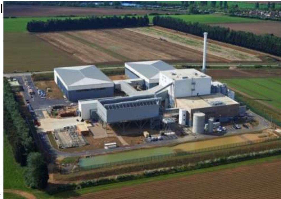
Sleaford straw-fired Renewable Energy Plant
